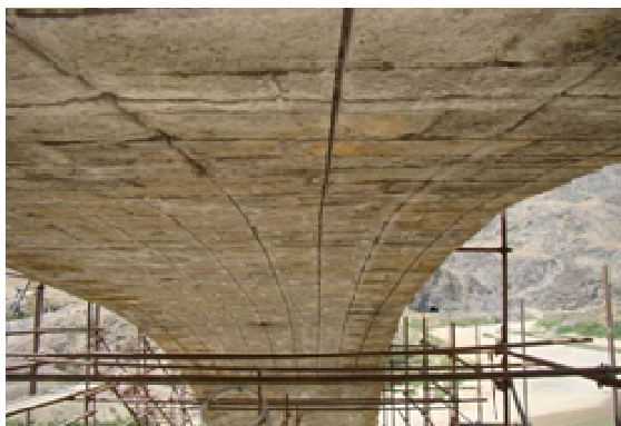
Fig. 31: Sub structural reinforcing of Ghaflankoh railway bridge on Tehran – Tabriz route (source Dez Ab 2011)
