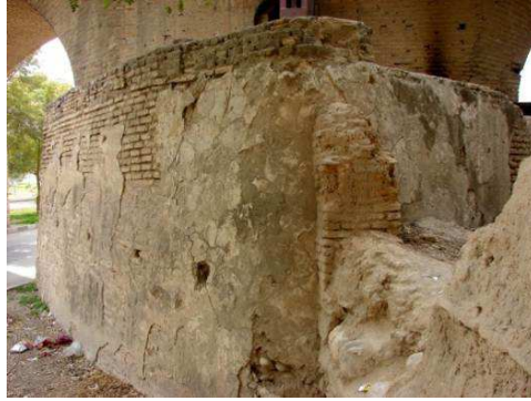
Fig. 8 Wall added to the flow breaker (2015)
