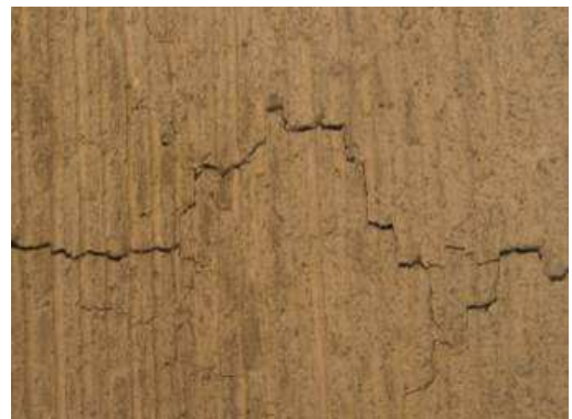
fig. 13 Cracking along the arch joints (2015)
