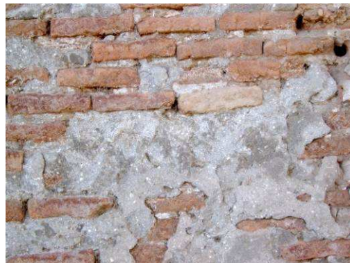
Fig. 7 Cement covering on historical brick (2015)
