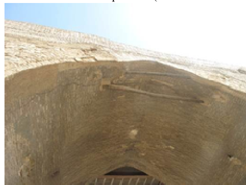
Fig. 28: Remains of scaffolding used for the repairing of the Structure( source the author-2014)
