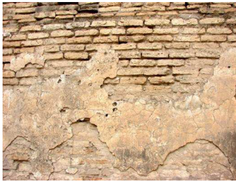
Fig. 9 The crumbling of the filling between the bricks and poor plastering (2015)
