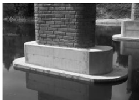
Fig 40: Creating a foundation underwater using an Underpinning method. (Source Dez Ab, 2011)
