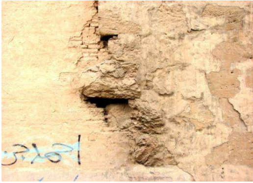
fig. 14 Separation between stone masonry and clay bricks (2015)
