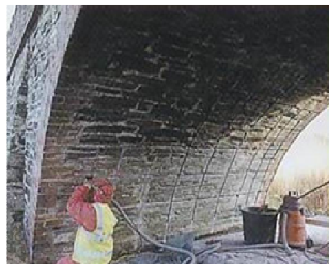
Fig. 32: Sub structural reinforcing using special winding steel rebars in stone and brick arches (source Dez Ab 2011)
