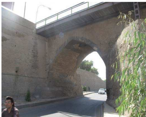
Fig. 25: Application of cement plastering to cover arch cracking ( 2015)
