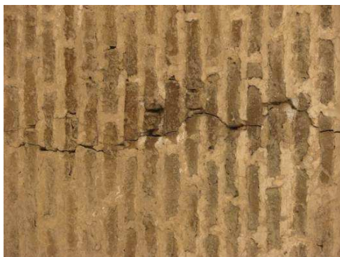
fig. 11 Cracking along the arch joints (2015)
