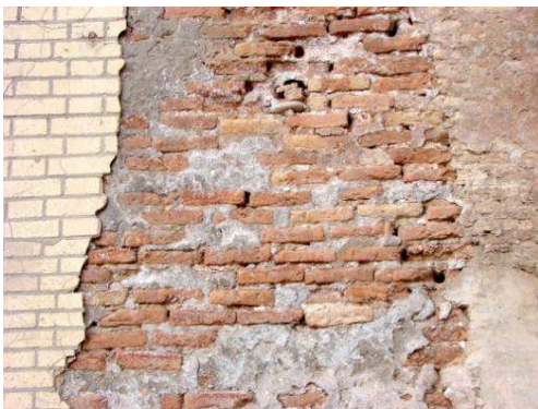
fig. 16 Cement covering with a brick design over the pedestal (2015)
