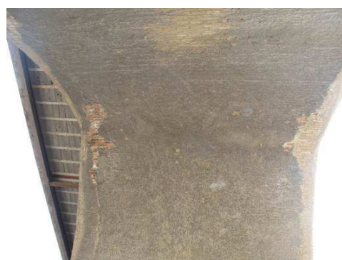
Fig. 26: Repairing of arch using abode brick and cement plastering in recent decades (2015)
