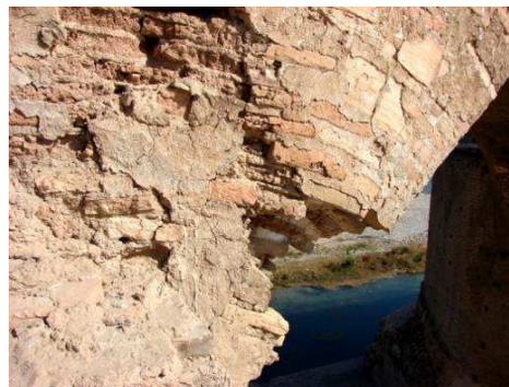
fig.22 Destruction of the arch foundations (2015)
