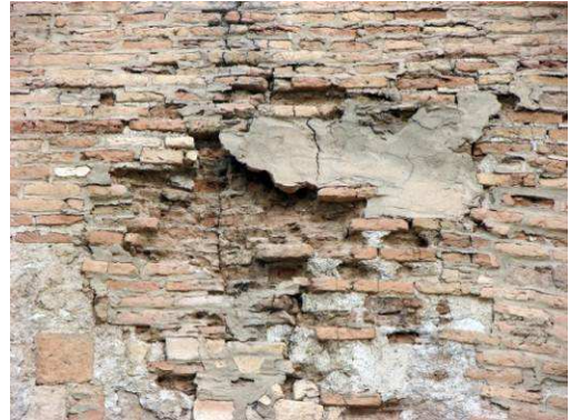
fig. 17 Damage due to the malfunctioning of the water conduit (2015)
