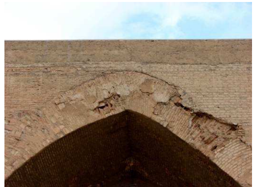
fig. 18 collapse of the upper part of an arch (2015)
