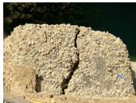
fig. 23 Deep crack in foundation (2015)
