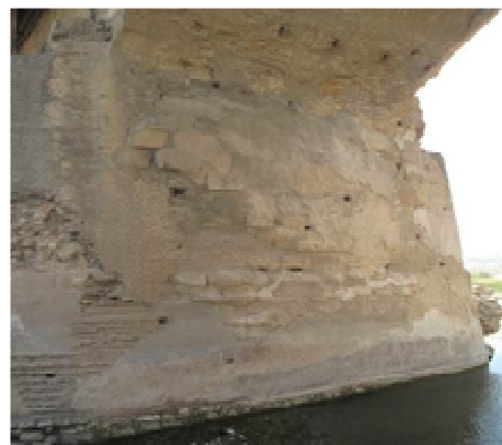
Fig. 27: Remains of scaffolding used for the repairing of the Structure over various periods (source the author-2014)
