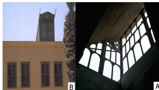
Figure 4. A- Internal view and B- External view of the Malqaf (Bahadori Nejad, Mahdi, Dehghani, Alireza, 2008).
