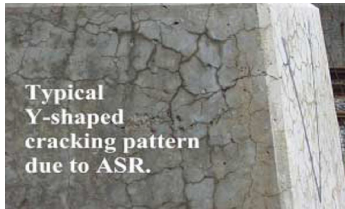
Fig. 1: Physical distress mechanisms of ASR [17].
