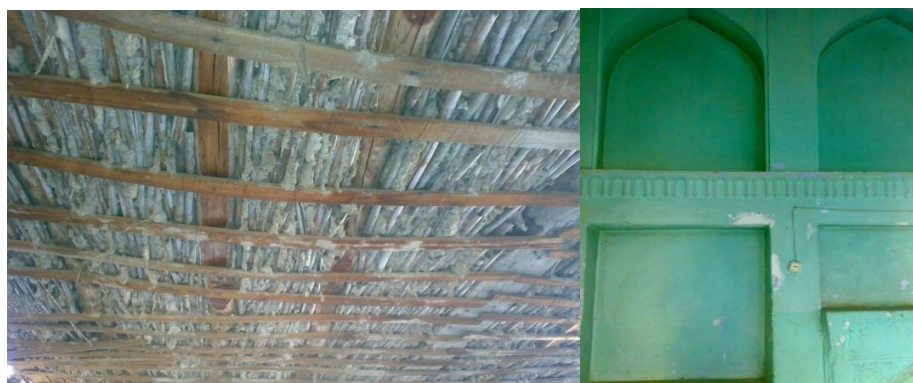
Ceiling coverage of stairs with puncheon, mud and reed available Shelves and arches inside building
