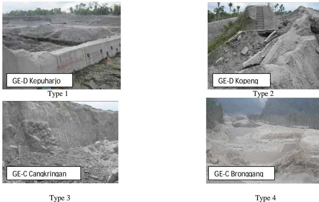
Figure 5: Example of each damage type in Gendol River
