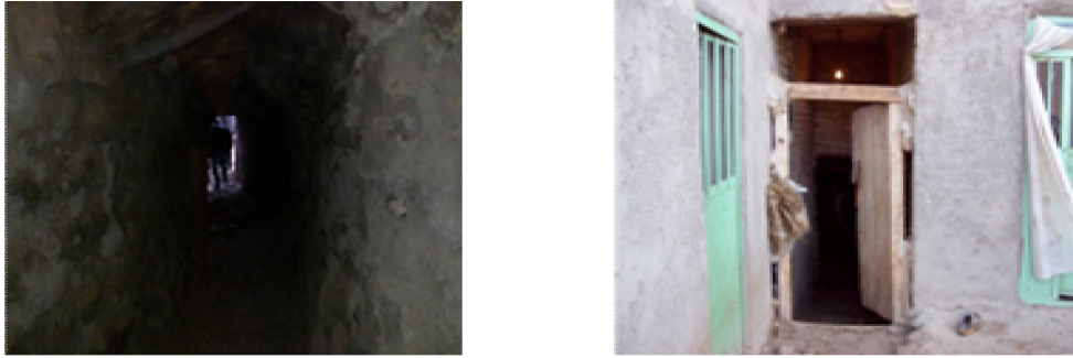
Fig.10. Kohul Entrance in a sample village house
