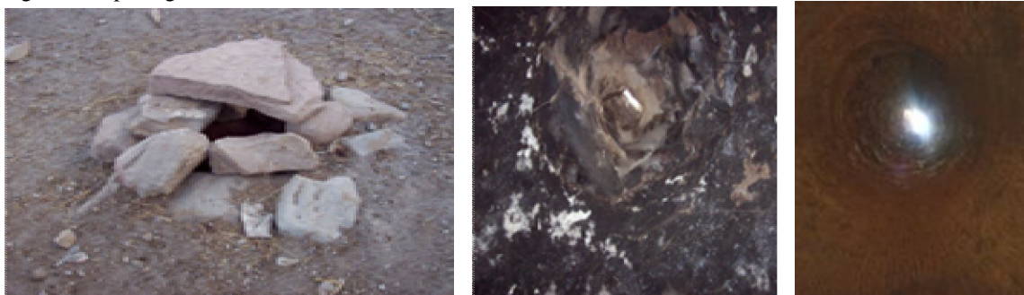
Fig.6. Kohul opening to provide light and ventilation
