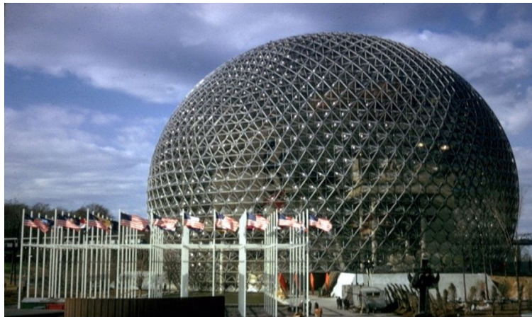
Figure 14: Use of space frame structure like geodesic dome picture for exhibition function, USA Pavilion, Expo 1967, Canada. [26]
