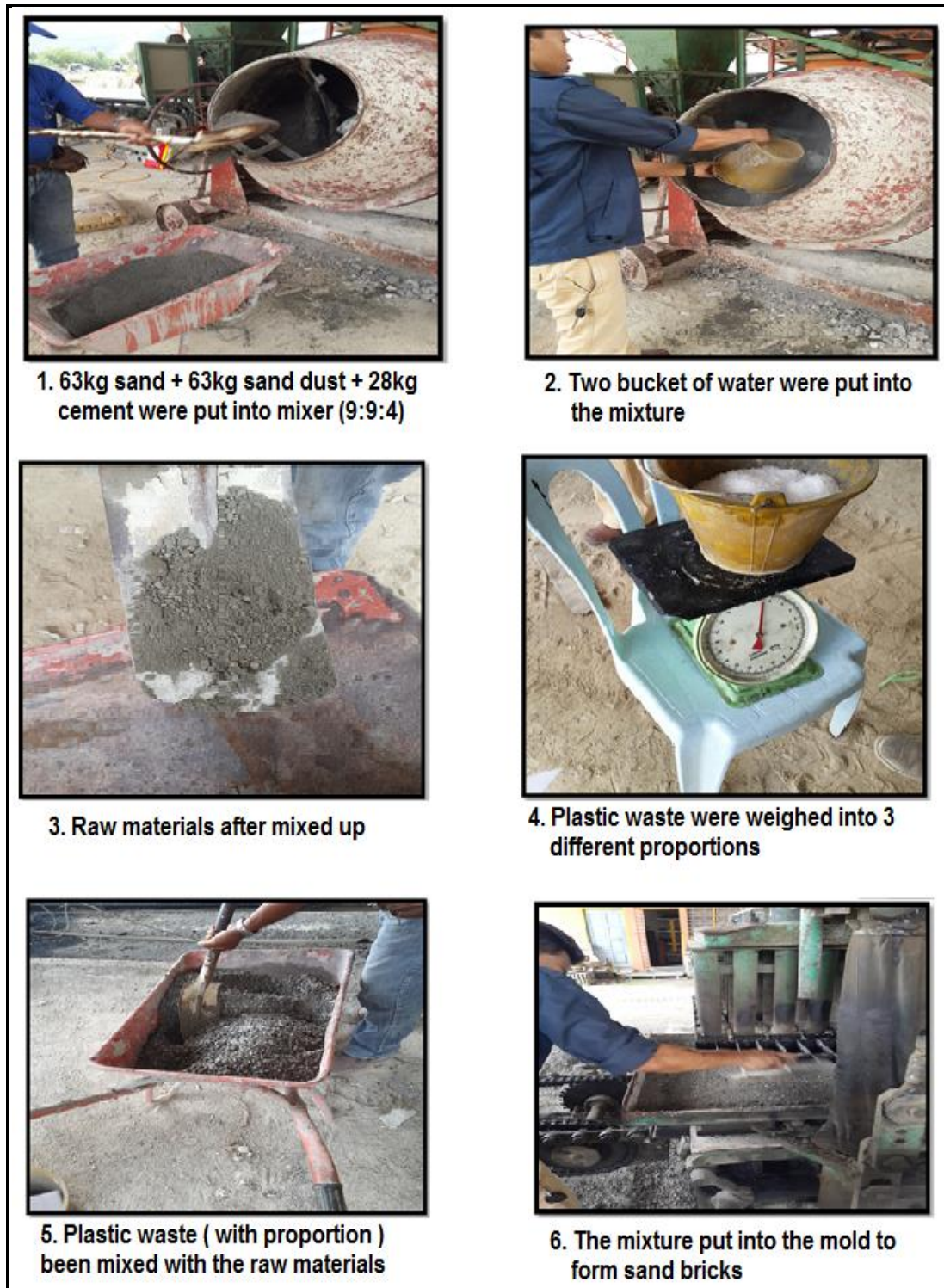
Figure 2: Sand bricks preparation
