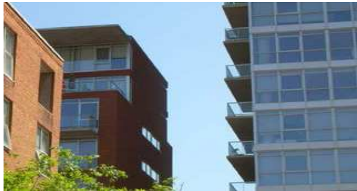
Fig. 6. Balconies rotation to reduce direct view to the neighbors[9].
