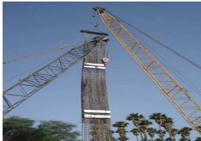
Figure (8) reinforcement baskets accompanied by mechanical joints
