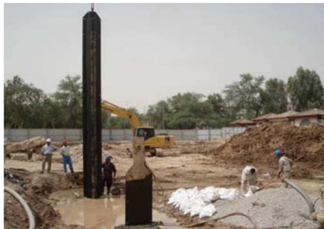
Figure(11) installation of stop end
