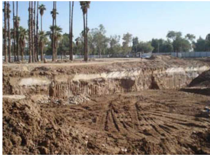
Figure (13) diaphragm wall of park station after excavation
