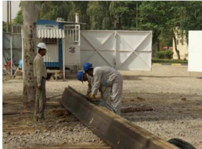
Figure (9) installing water stop inside the Stop end
