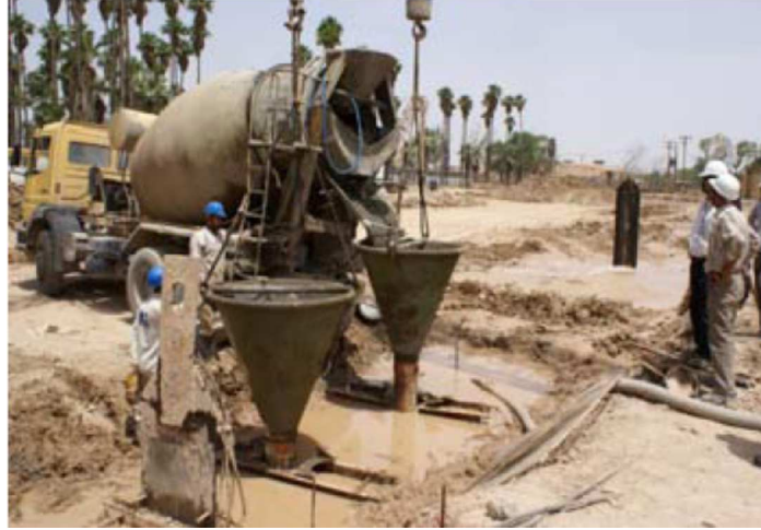
Figure (12) concreting of diaphragm wall by shoot and two tremie pipes
