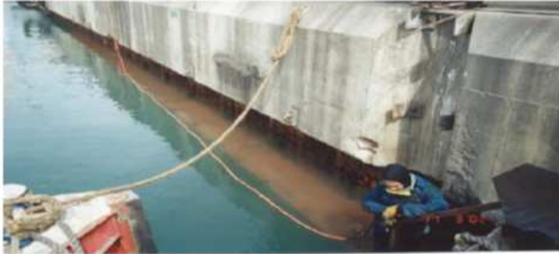
Fig.2. The lower part of the formwork is mounted to sheet piles
