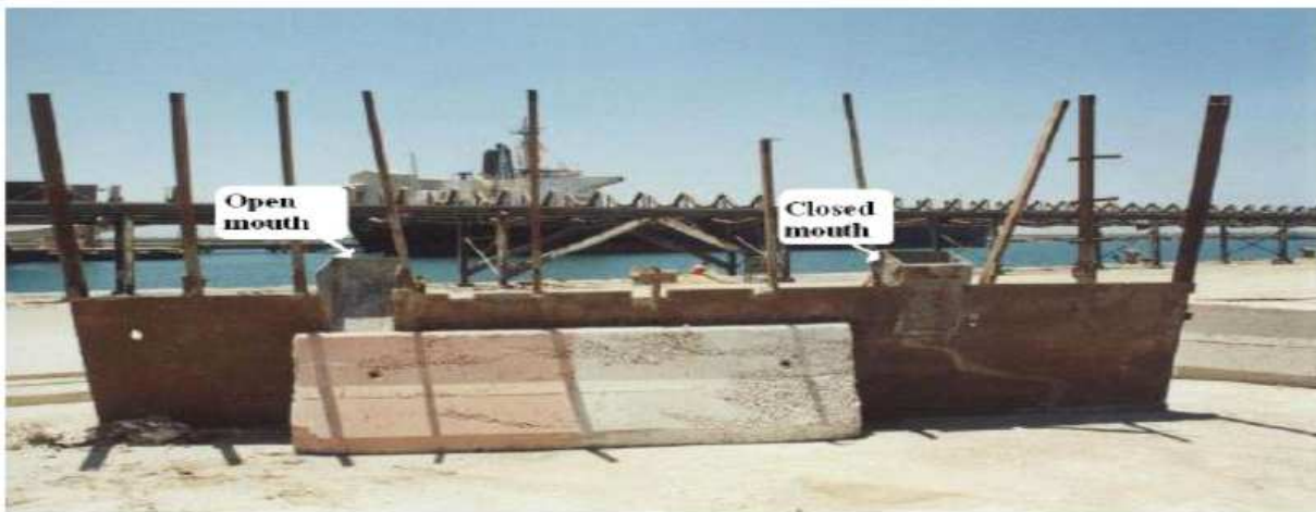
Fig.3. The upper part of the formwork is mounted to sheet piles
