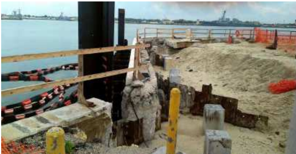
Fig.6.Photo of Partially Excavated Cell with Upper Deck Foundation Piles.
