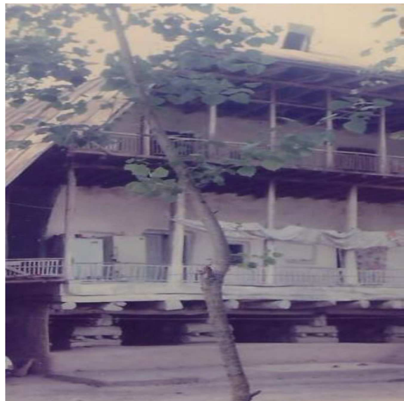
Picture 2. General façade of a traditional building on the basis of Lahijan's wooden rollers foundations
