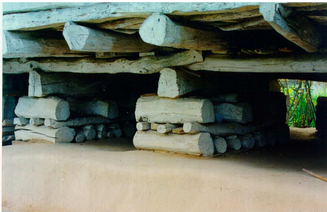
Picture 3. Façade of wooden rollers foundations
