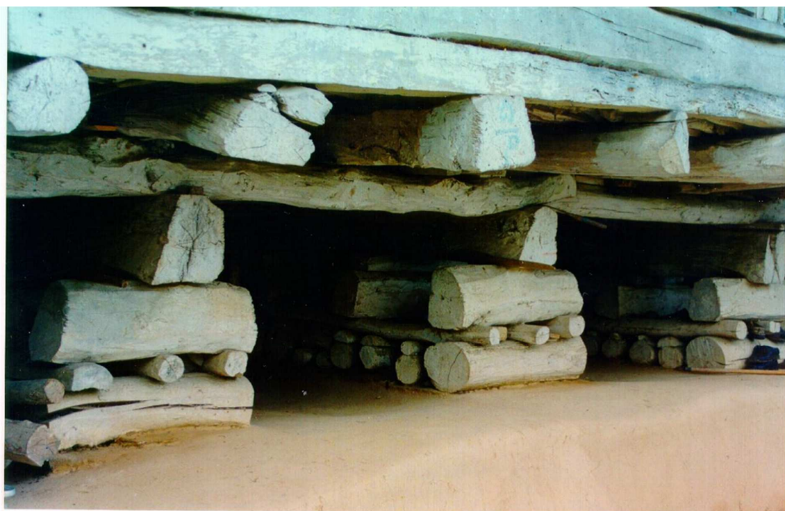
Picture 4. Façade of wooden rollers foundations
