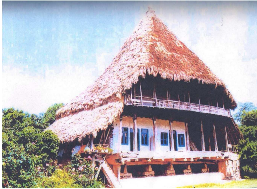
Picture 1. General façade of a traditional building on the basis of Lahijan's wooden rollers foundations
