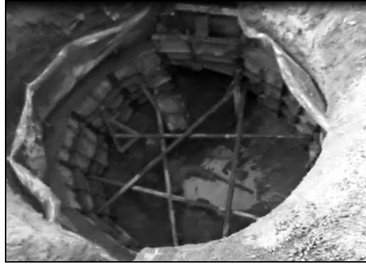
Fig.6. Initial stages of reactor concreting
