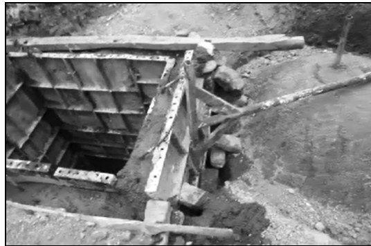
Fig.7. Final stages of reactor concreting
