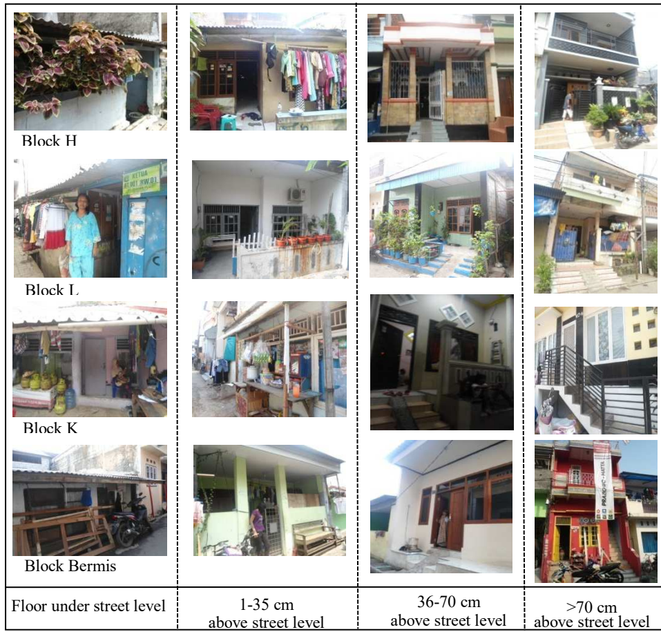
Figure 4. The elevation of ground floor: from “very vulnerable to flood” to “the safest from flood”
