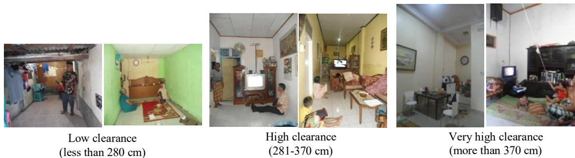
Figure 5. The ceiling conditions: from “low clearance” to “very high clearance”
